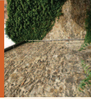
Fig. 52 Limestone tenement and outbuilding walls located west of St Aldates.
