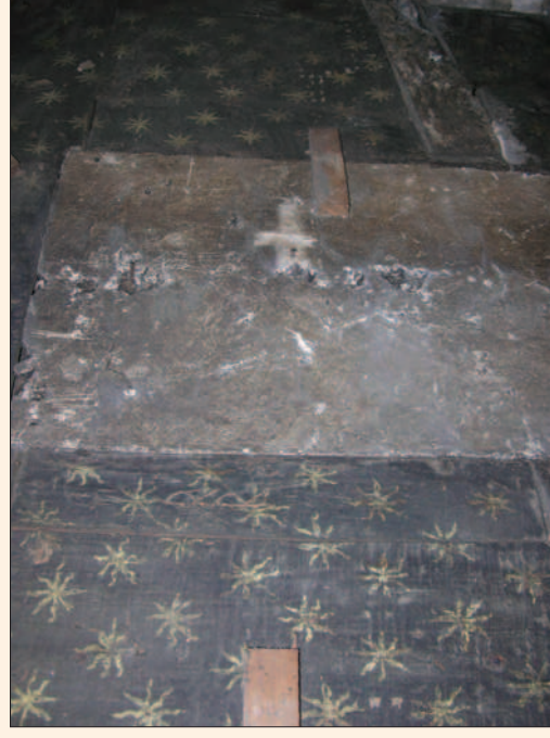
Fig. 30 Painted panelling and a door from a previously unknown 17th or early 18th century student study exposed at Brasenose College during building work in 2010.
