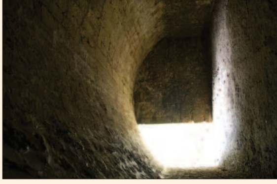
Fig. 28 A vaulted cellar and entrance chamber discovered in 2009 during building works at The Queen's College. Dated to the 17th century but perhaps containing fabric of earlier origin.
